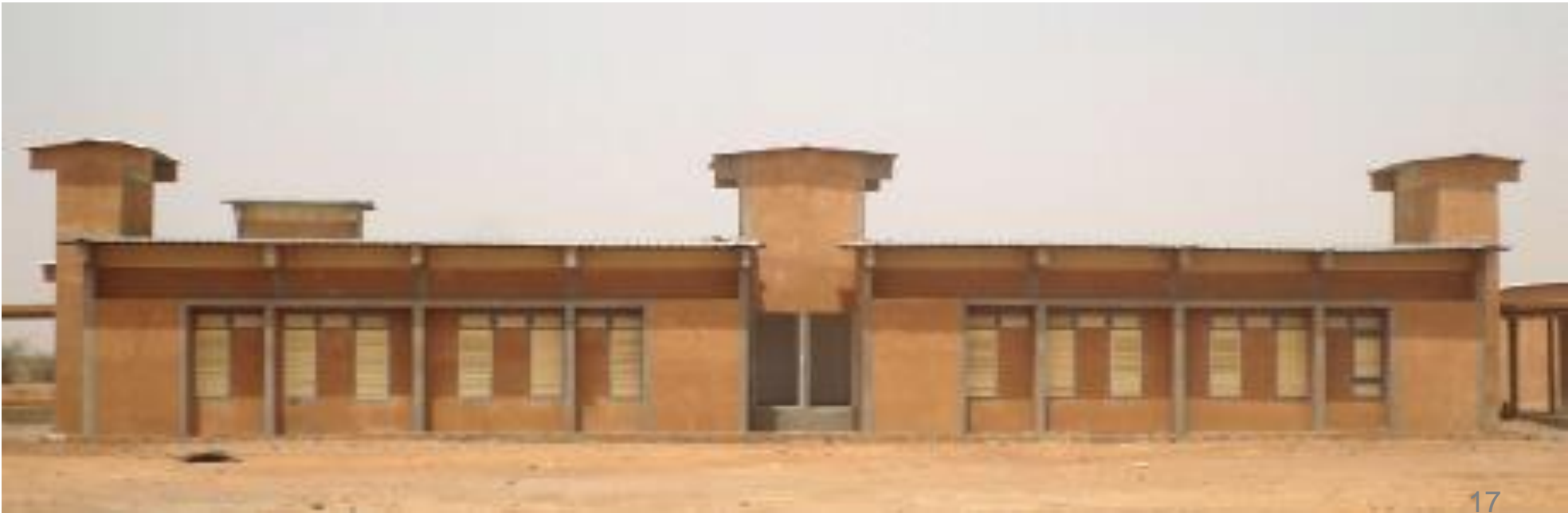
Solar chimney, Luxembourg Cooperation in Niger, 2016
