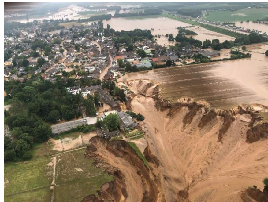
Flood damage in Erftstadt-Blessem in Rhein-Erft-District of Germany. 17 July 2021
